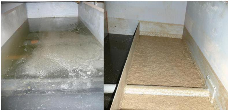
Gas bubble and floc production in flotation/sedimentation tank
